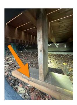
Structures over 24" in height should have 10" (diameter) concrete pilings that extend below the frost line. At the time of the inspection, it was undetermined if these pilings existed with the structure. This should be further inspected and corrected if needed.
