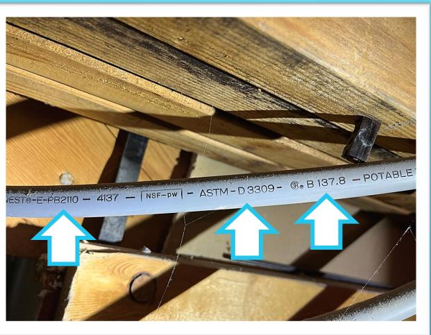
POLY-B WAS THE SUCCESSOR TO COPPER WATER PIPING WHICH LED TO GREAT DESIGNS SUCH AS HOME-RUN MANIFOLDS (THIS RESULTED IN CONTINUOUS PRESSURE FOR YOUR SHOWER) AMONGST OTHER ITEMS. UNFORTUNATELY, THE MATERIAL WAS PROBLEMATIC FOR A VARIETY OF REASONS WHICH LED TO FAILURES IN SOME INSTALLATIONS. DEPENDING ON THE AREA, TYPICALLY POLY-B WAS FOUND DURING THE MID 1980S – TO MID 1990S.
